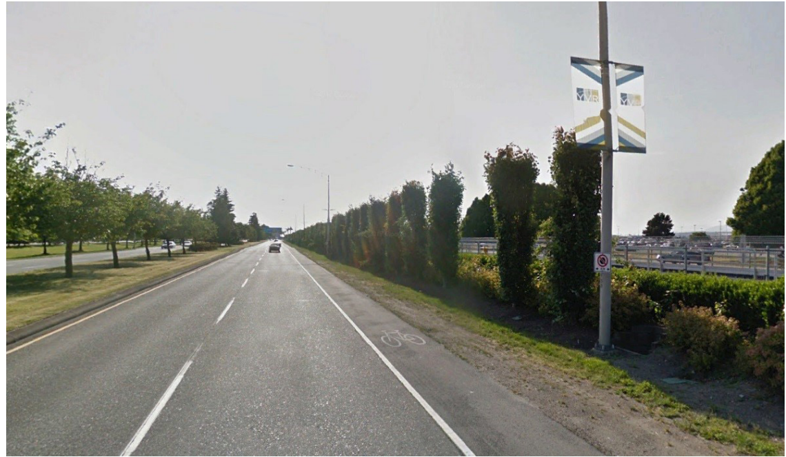
Figure 2.6ae: Dedicated Bike Lane Connection
